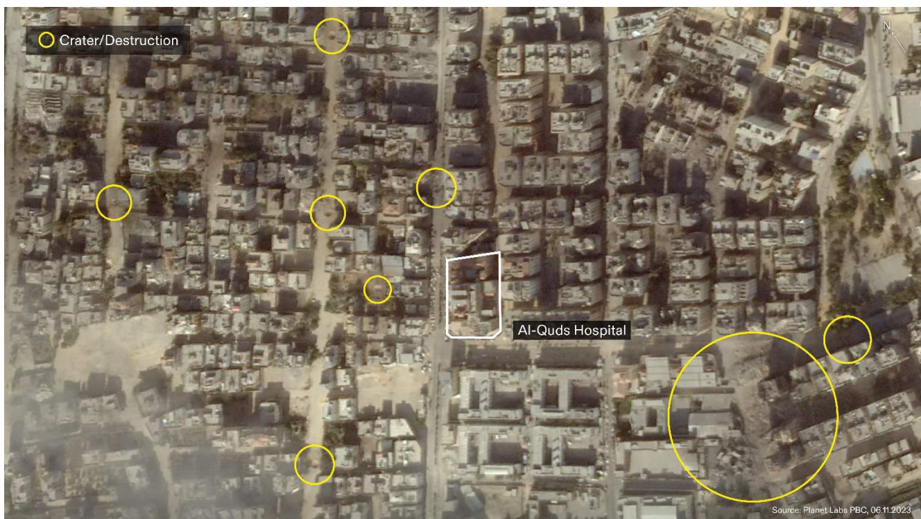
Figure 12: Satellite image of Al-Quds hospital. In yellow, craters and destruction areas caused by strikes on the main roads surrounding the hospital.
